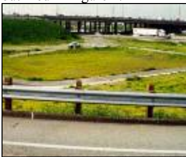
Figure 1. Example of an Infiltration Basin
