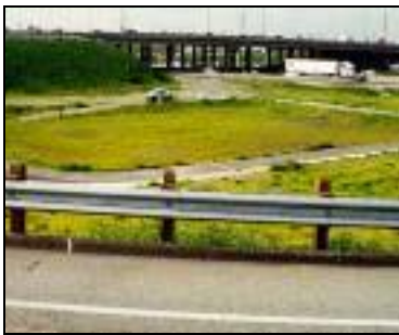
Figure 1. Example of an Infiltration Basin
