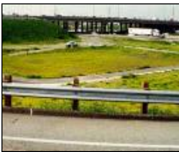
Figure 1. Example of an Infiltration Basin
