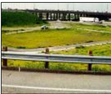
Figure 1. Example of an Infiltration Basin.
