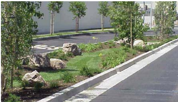
Figure 1. Example of a Linear Bioretention Area Photos: Los Angeles Basin Water Augmentation Study – Neighborhood Retrofit Concept Plan
