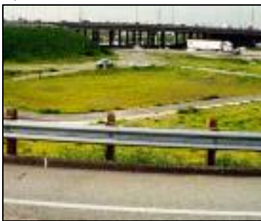
Figure 1. Example of an Infiltration Basin
