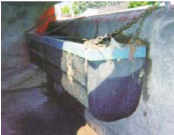
Figure 1. Catch Basin Insert
