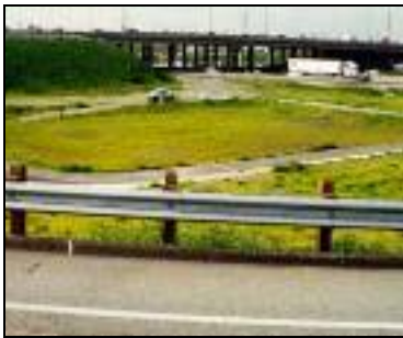
Figure 1. Example of an Infiltration Basin
