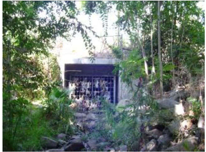
Figure E-44. Stormwater outfall at the end of Rush St.
