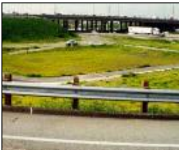
Figure 1. Example of an Infiltration Basin
